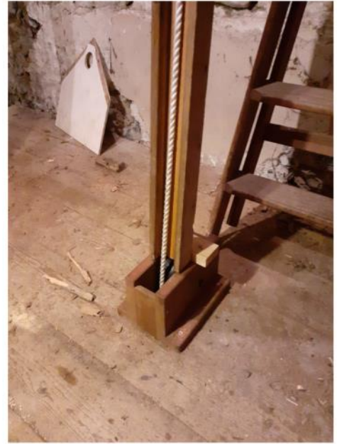
New wide pulley (to accommodate sally of 6th that comes through clock room floor).
