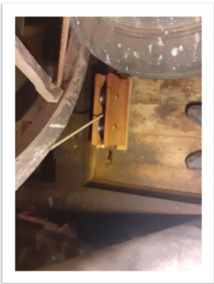
New double pulley of 6th in the belfry beside the old hole elongated by rope wear
