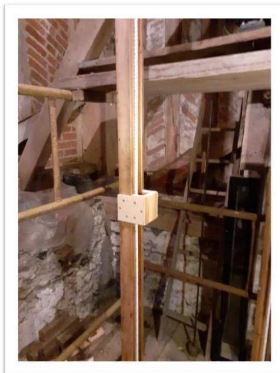
Clock room showing bridge on rope chute to inhibit the formation of a standing wave
